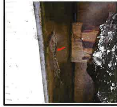
Photo A-39: Delamination on the bottom of the concrete slab at beam 13-4.
