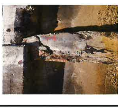
Photo A-46: Delamination at the bottom of the concrete slab between beam 14 and beam 14-4.
