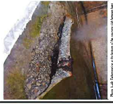
Photo A-39: Delamination on the bottom of the concrete slab at beam 13-4.
