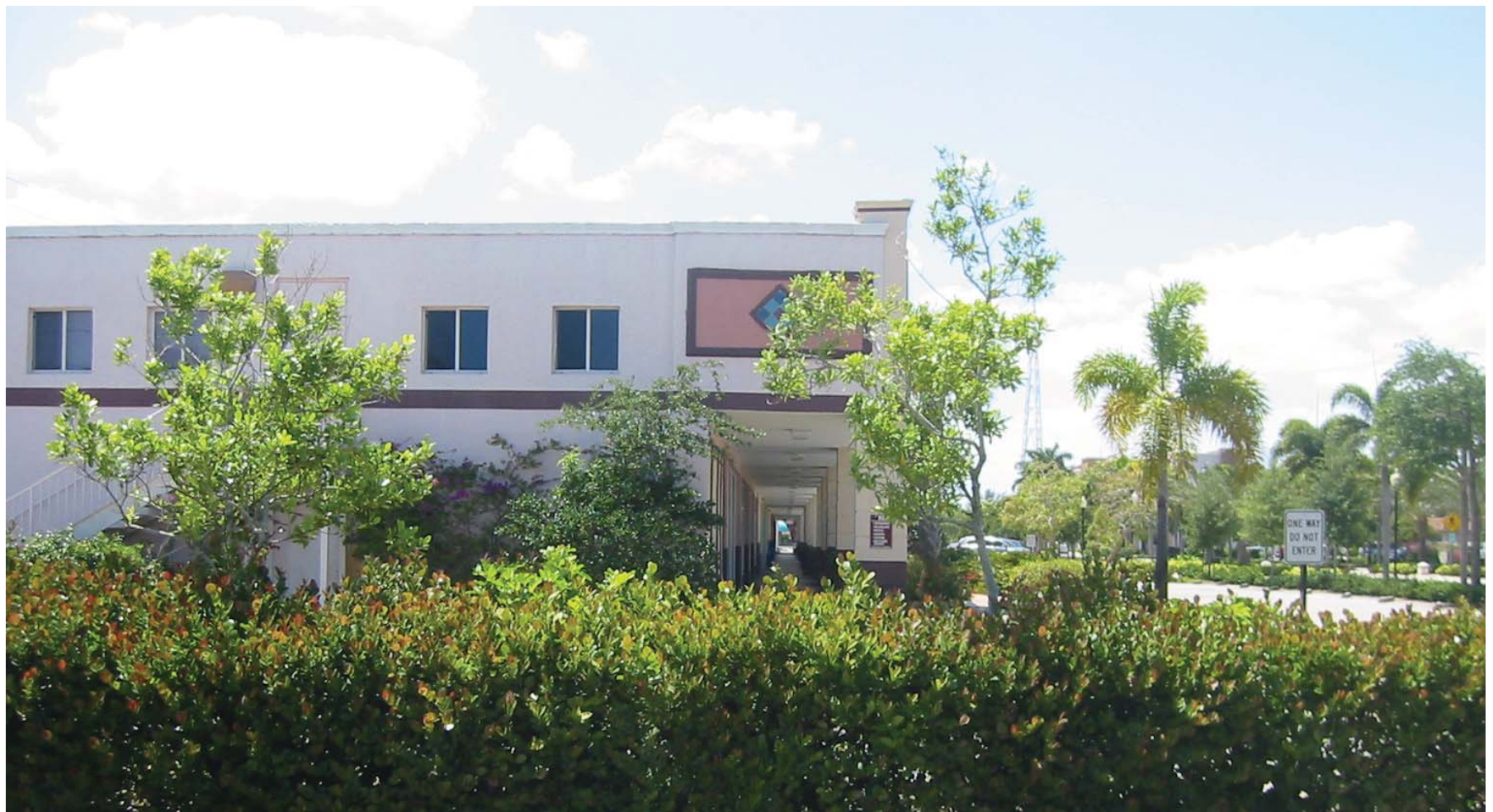
Interrupted pedestrian connection between the sidewalk and the building. Strategies are discussed in “Recommendations”
