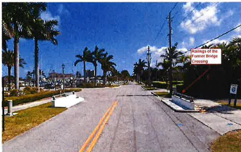
Existing Former Bridge on Lake Shore Drive
