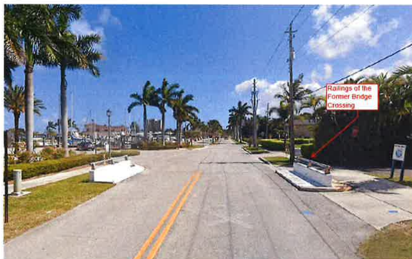
Existing Former Bridge on Lake Shore Drive
