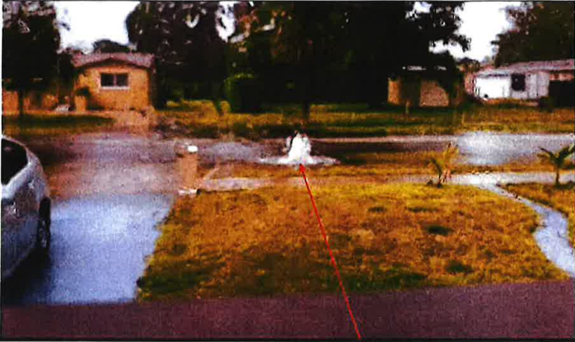
Backflow surging from pipe
