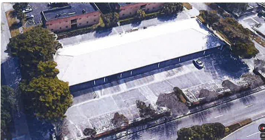
Figure 2: Panoramic view of site, looking east from 10 th St.
