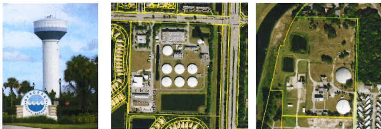
Photo 1: SUA Water Tower Hood Road Facility; Photos 2 and 3: Aerial view of Richard Road and Hood Road Water Plants 2018
