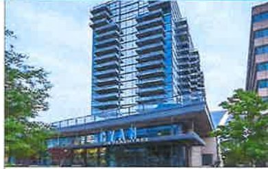
High rise buildings (up to 20 stories)
