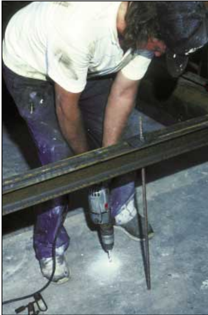
Figure 76 Inside the house, workers drill holes in the concrete slab ...
