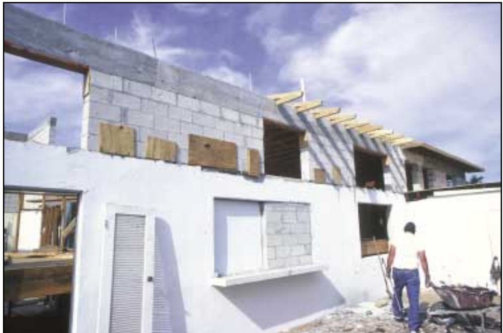
Figure 67 The extended first-story walls.
