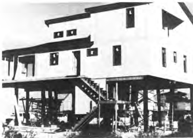
Figure 4.14. Pile Foundations
