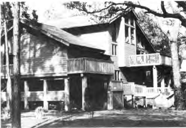
Figure 4.3. Elevation by Posts
