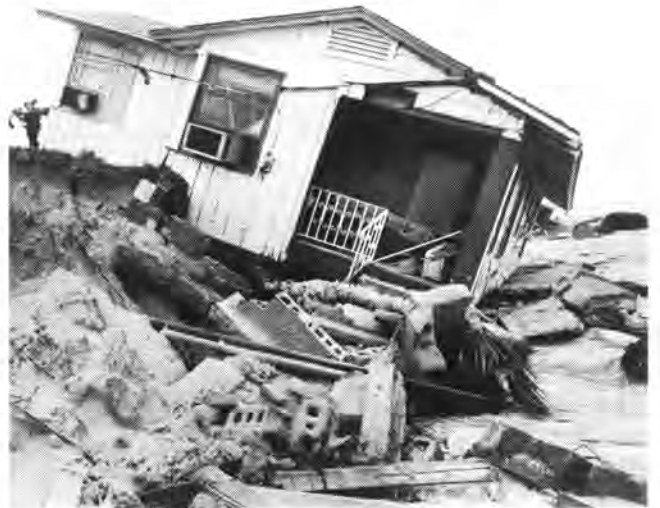
Figure 2.3. Erosion Caused This Foundation to Collapse.
