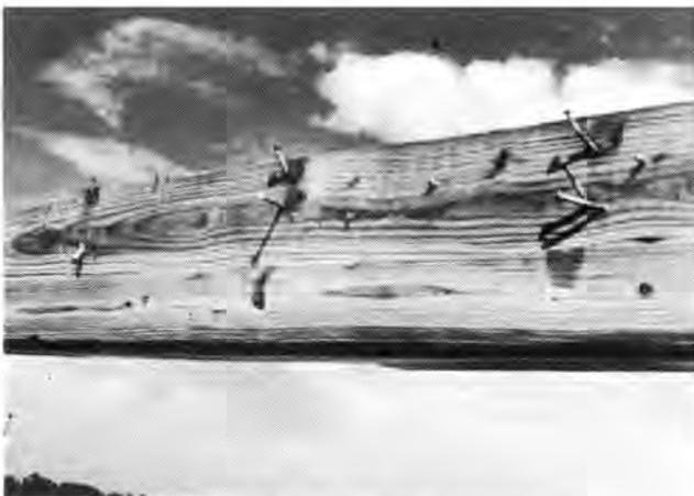
Figure 4.26. Toe Nailing Provides Limited Pull-Out Resistance
