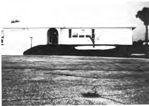
Figure 4.1. Elevation by Earth Fill
