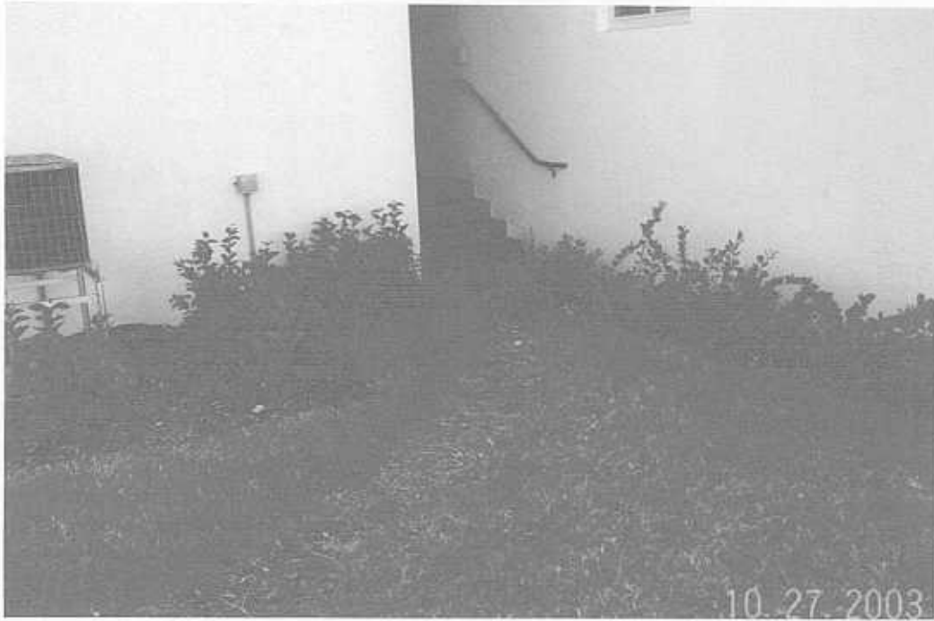
North stairwell on Building 1 Type IV
