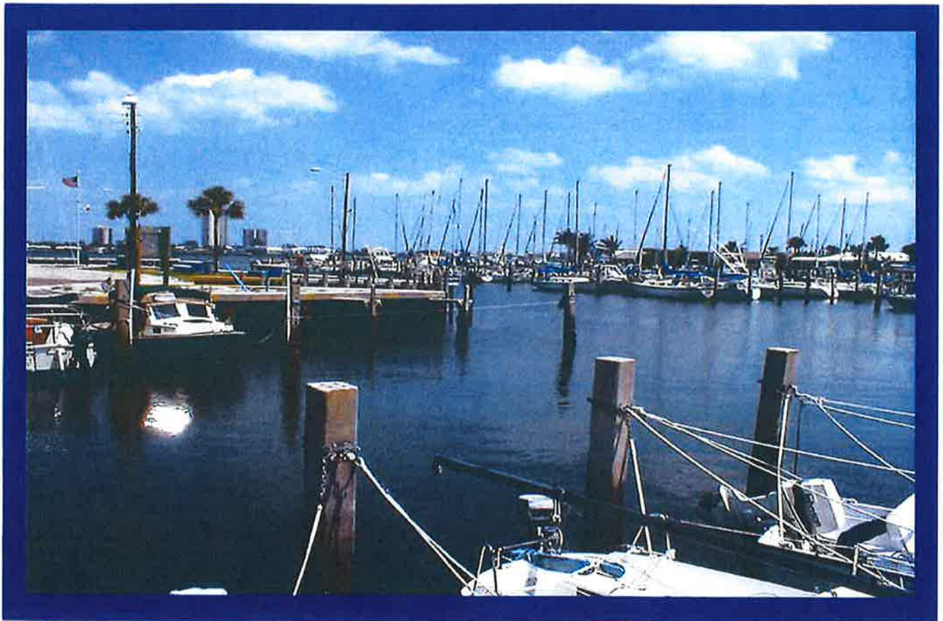
Marina To Be Renovated By The Town of Lake Park
