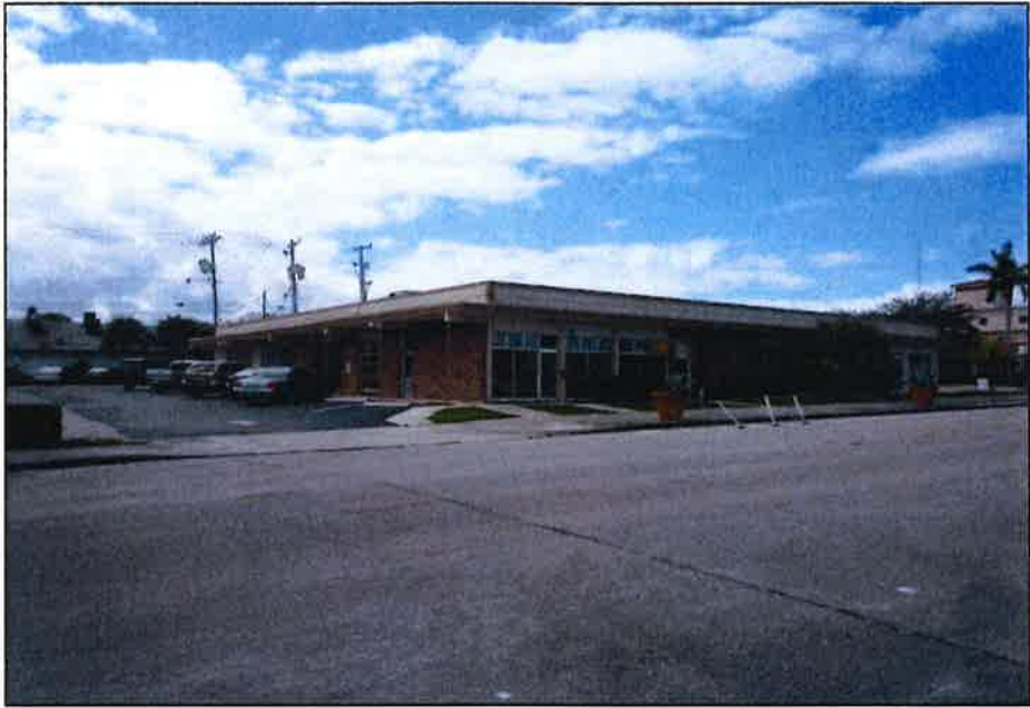
North and east side of subject
