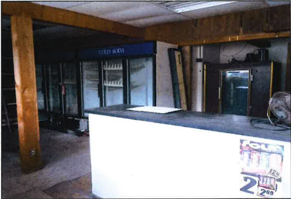
Interior of Unit 101 (former liquor store)
