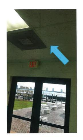
After investigating the source of all the leaking. It comes down to the delamination of the stucco at the transition point between the second floor balcony and the first floor exterior wall. This gap is allowing water to seep behind the wall. It is then finding it's way between the tongue and grove joints in the second floor concrete planks and ultimately this water is ending up getting into the interior spaces of the building.
