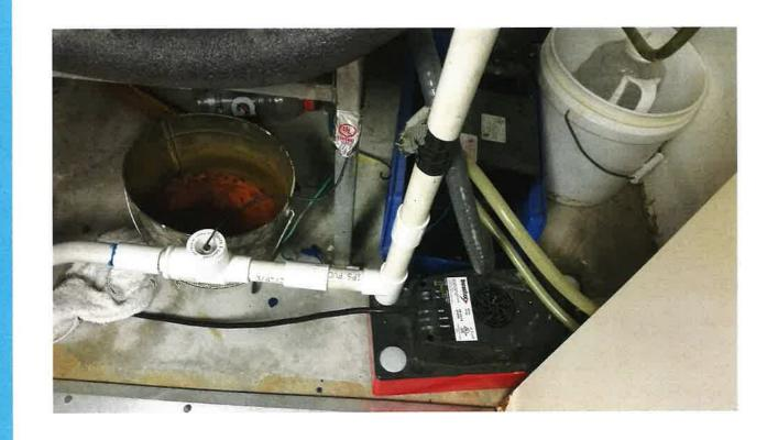
Drain is in the wrong place in the elevator shaft. It is located 4 inches from the bottom of the elevator shaft, on the wall. Instead, it should be in the floor, so there will not be any standing water in the elevator shaft well area at all. This is causing safety issues with the mechanical operations of the elevator.
