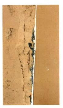
As you move around the building you will see a lot of cracks in the stucco. Some of the cracks are repairable and a lot of them are not, which will require the stucco to be replaced.
