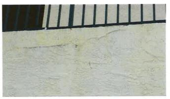
Continuing to move around the building clockwise, you will see more cracks in the stucco on the south side of the building.
