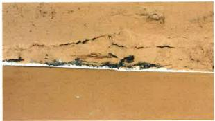
Some more pictures showing the delamination of the stucco and concrete at the edge of the second floor balcony.
