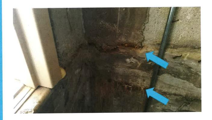
Between the water coming in from the second floor concrete, it is also coming from under the doors themselves. This water has cause the elevator to have safety issues with the rusting of the high pressure pipes for the elevator. Which could cause a lift failure and the possibility of a free fall dropping of the passenger compartment.
