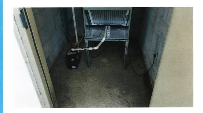
No drain for the ship's store HVAC unit either. It also is using a sump pump to pump the AC condensation up to second floor to get rid of it's water.
