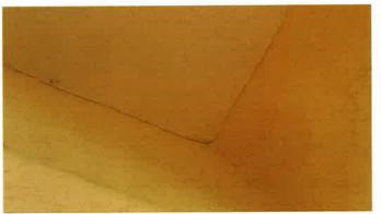
There are cracks on the second floor balcony running in different directions in that same area. There is a pop in the tile next to a column in the men's bathroom. It is like that part of the building is floating up and down, because the pilling that is not installed correctly.
