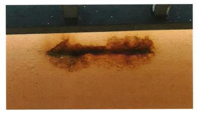
Most of the handrail post needs to be filled in and sealed.
