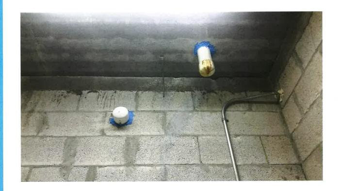
No drain for west wing first floor HVAC unit. A sump pump is being used to pump the AC condensation up to second floor to get rid of the water. If you notice the damp floor, the sump pump does not a good job of moving the water, and the floor gets wet from time to time.
