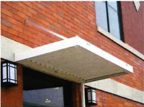
LOADING AREA CANOPY
