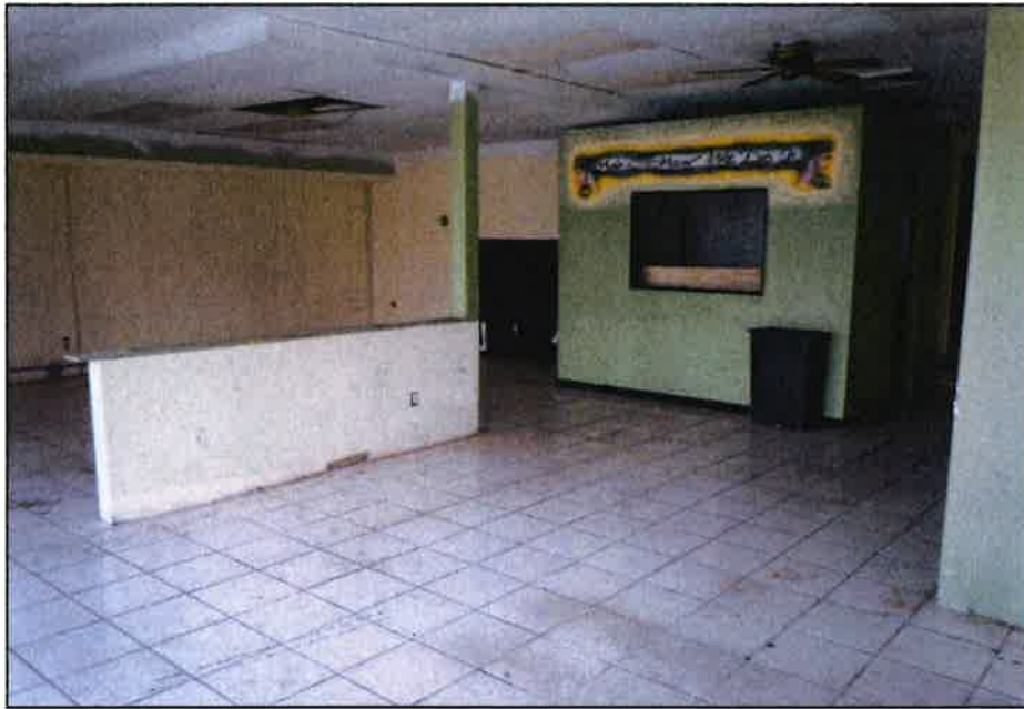
Interior of Unit 102
