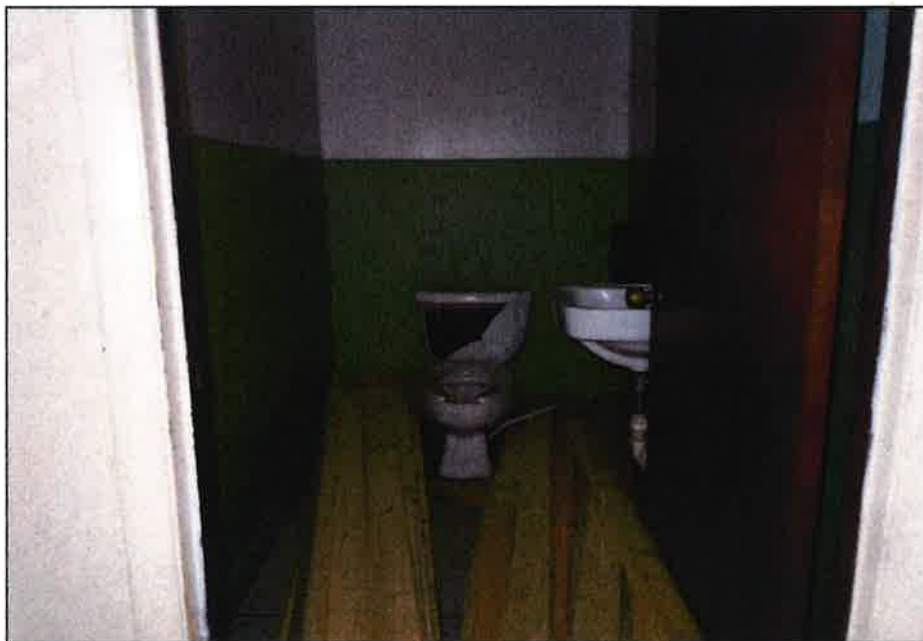
Interior of Unit 102
