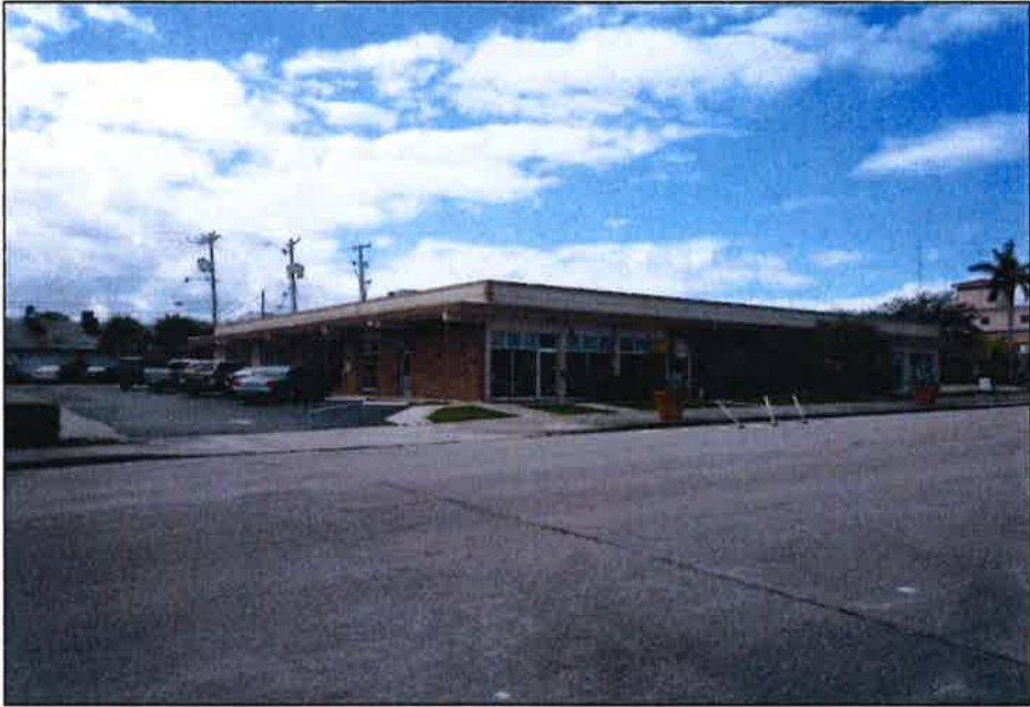
North and east side of subject
