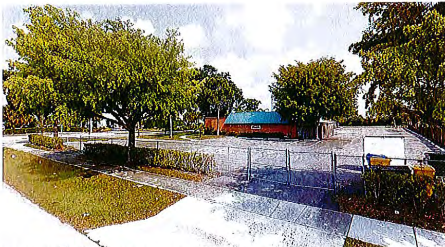
Illustrates the third point of access which is currently closed off by the existing fence. The picture also illustrates the rear parking area.
