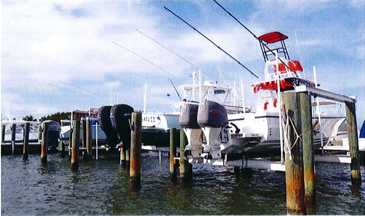
Photo - 10: Blowing Rocks Marina North side
