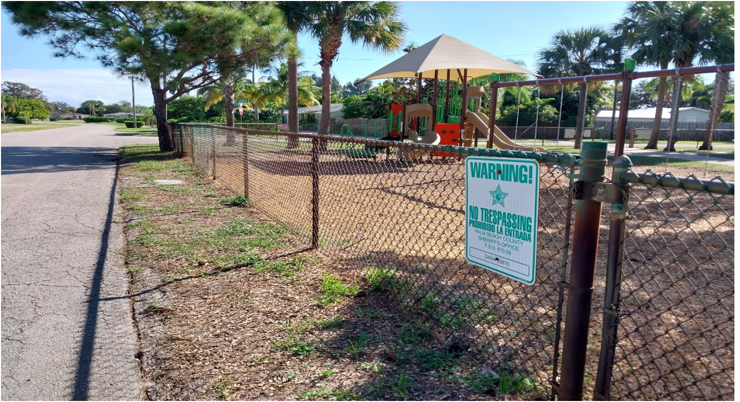
View of existing 4' high chain-link fence at perimeter of park
