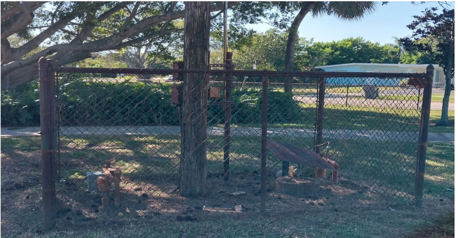
View of existing 6' high chain-link fence enclosure at electric / pump equipment
