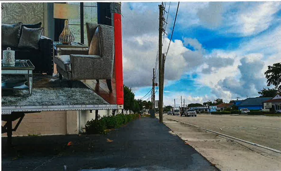
Photo: Faulty lot layout. Blank wall facing main street with no use zone adjacent to sidewalk.
