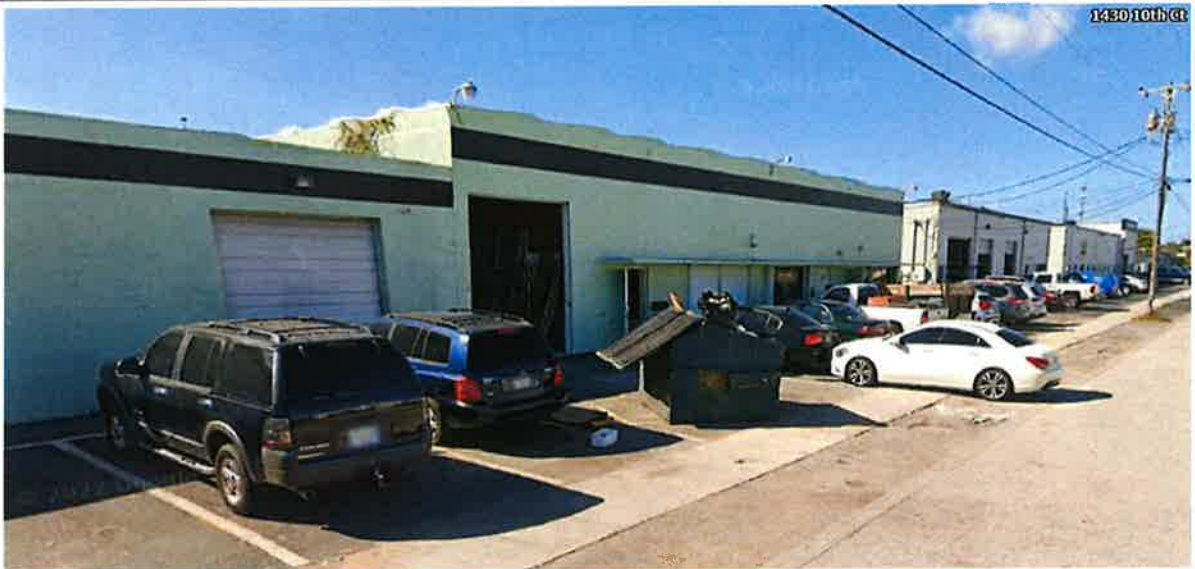
Photo: 10th Court deterioration of site improvements/ outdated building
