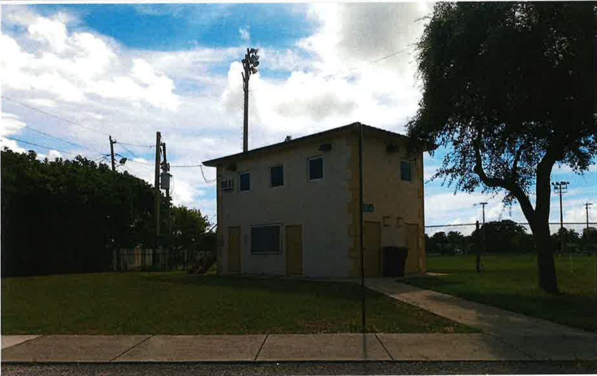
Photo: Silver Beach inadequate and outdated building at Bostrom Park
