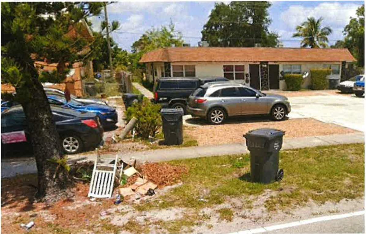
Photo: Silver Beach deterioration of site improvements
