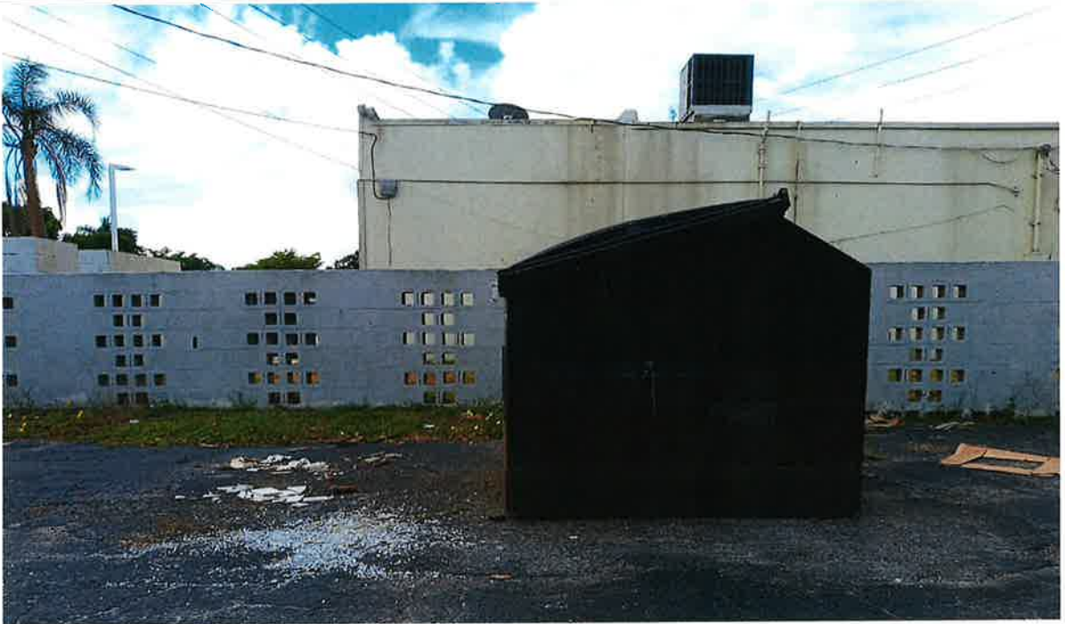
Photo: Broken glass unsafe conditions.
