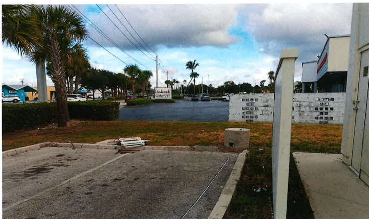
Photo: Faulty lot layout. Missing internal connections.
