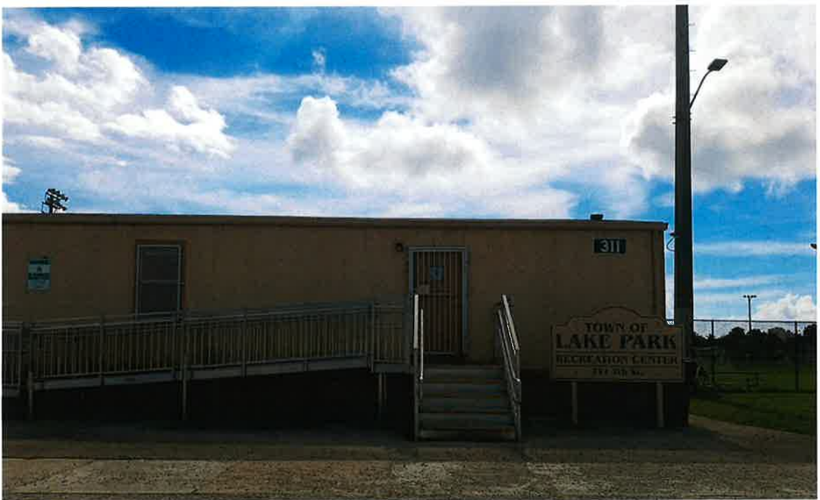
Photo: Silver Beach inadequate and outdated building at Bostrom Park
