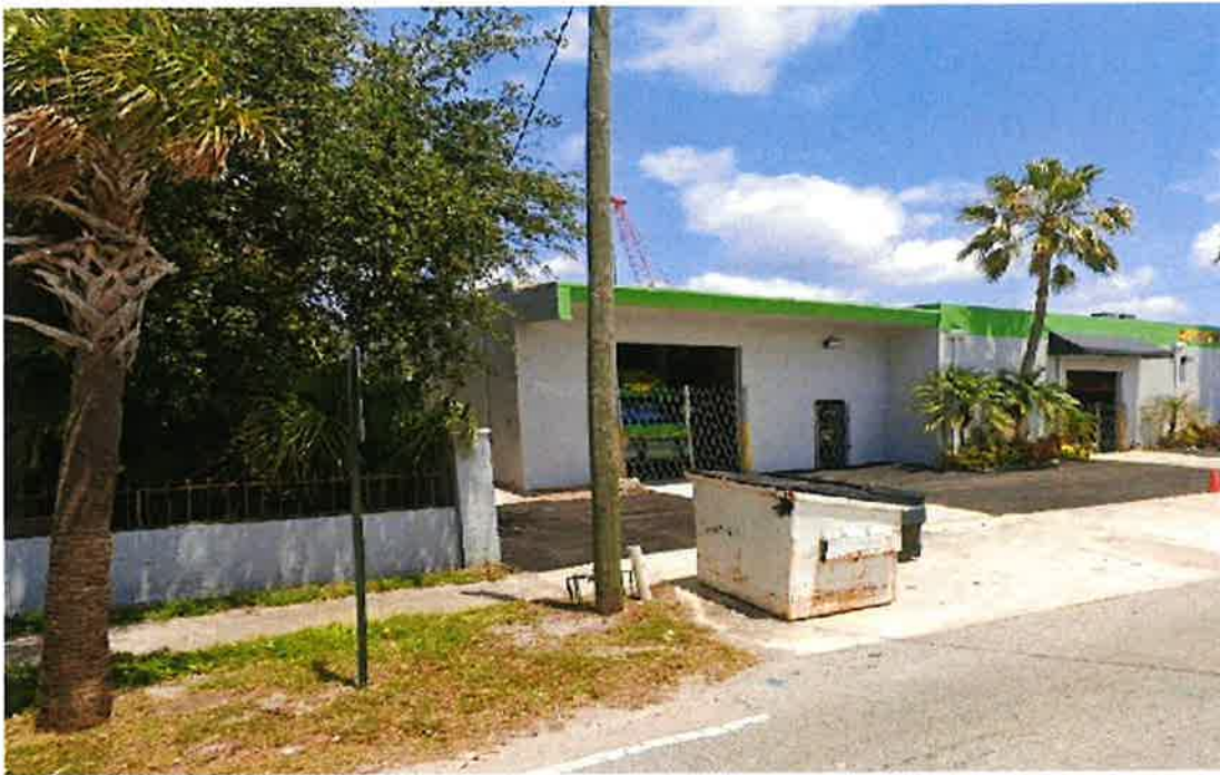
Photo: Silver Beach exposed dumpsters unsanitary conditions
