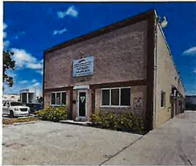
Figure 2 - 1343 S Killian Before Repainting
