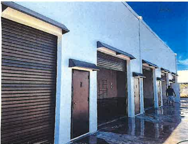
Figure 4 - Repainted 1343 S Killian Building Detail
