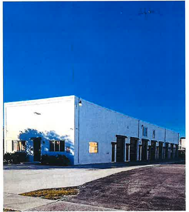
Figure 4 - 1343 S Killian Front Facade
