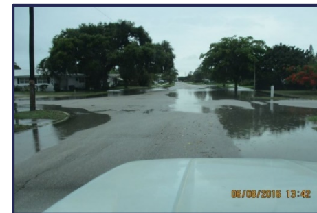
Lack of Drainage 2 nd Street Corridor)
