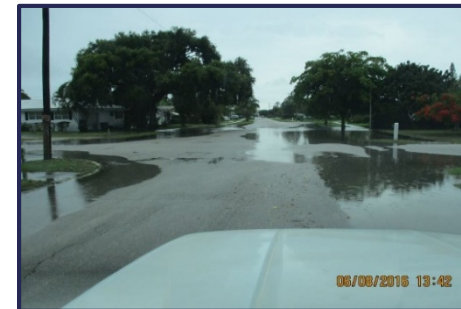
Lack of Drainage 2 nd Street Corridor)
