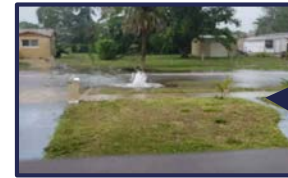
Ilex Court Inlet Surcharge
