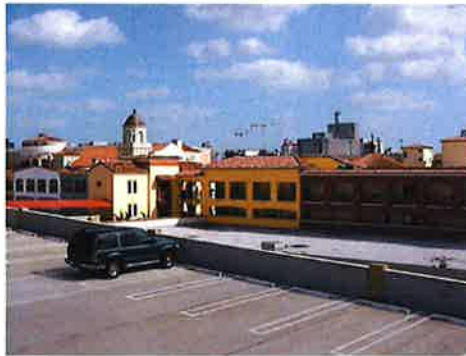
View from rear of lot showing parking garage structures lined along the street
