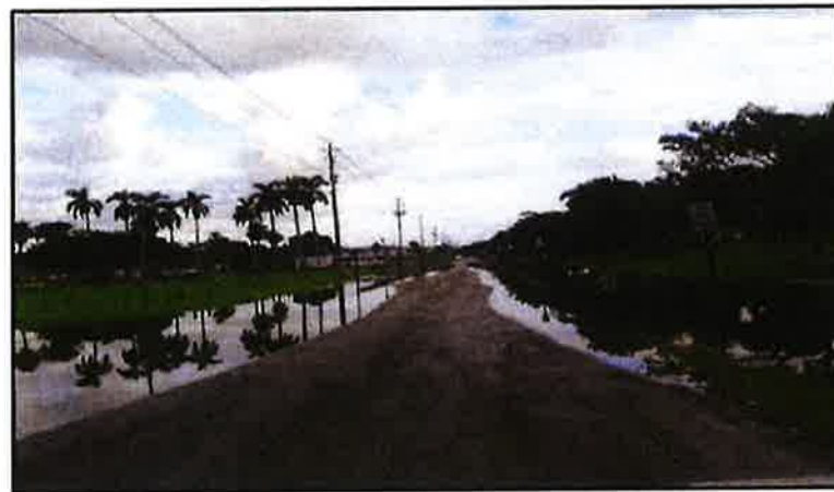
Figure 5-8 High Tide (SLR) Flooding Along Lake Shore Drive
