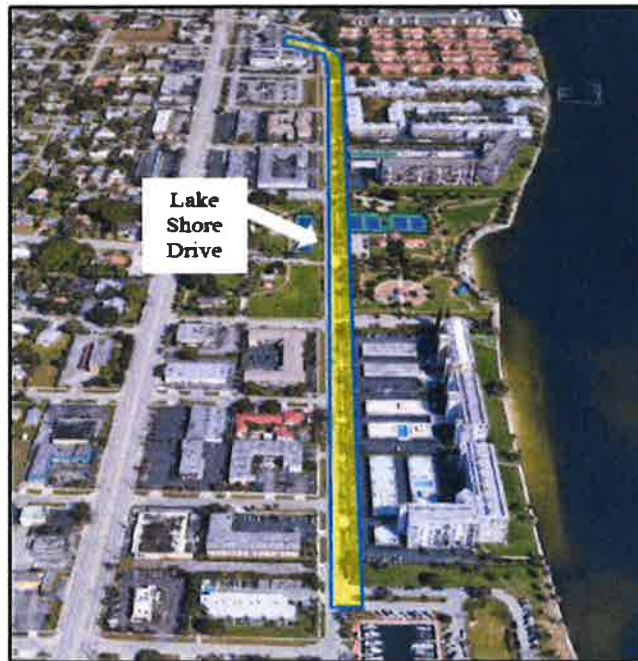
Figure 5-31 Lake Shore Drive Drainage Improvement Project
