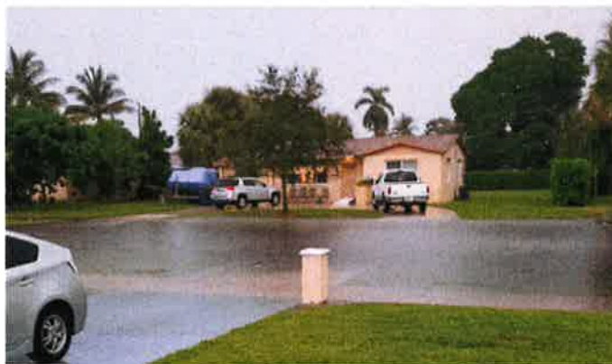
Figure 5-6 Inlet Surcharge at Ilex Street
