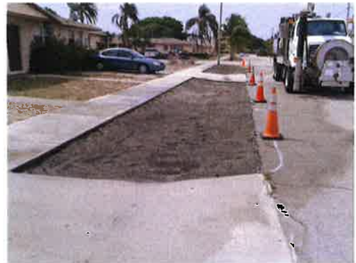
Figure 1. Typical swale before sodding.
