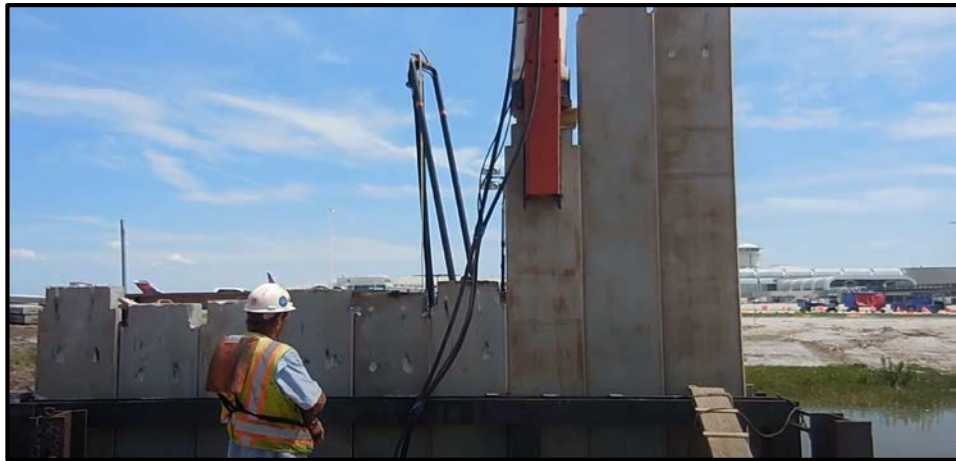
Concrete Sheet Pile Bulkhead
