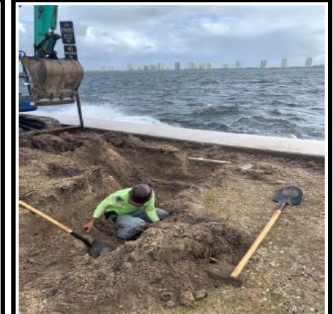
Photo A-69: Excavation Location 1 at Exhibit 1, Section 2, station 1+35.
