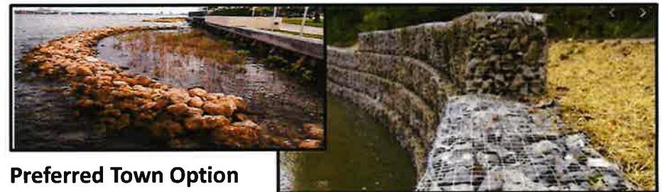
Combination Gabion Bulkhead & Living Shoreline
