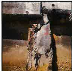
Photo E-48: Close-up of a vertical pile at the easement bulkhead.
