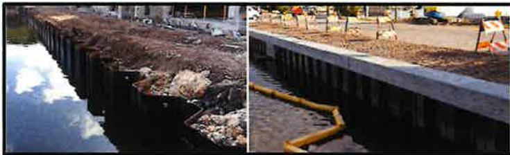
Steel Sheet Piles Bulkhead
