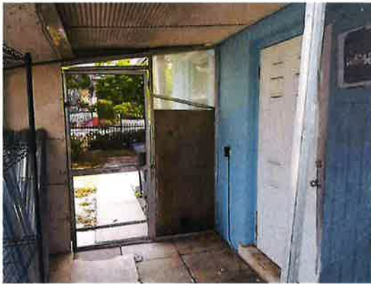
Scr.Pch Interior View
