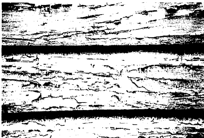
Fig. 9 Cracking, alligating and flaking are evidence of long-term neglect of painted surfaces. The remaining paint on the clapboard shown here can be removed with an electric heat plate and wide-bladed scraper. In addition, unsound wood should be replaced and moisture problems corrected before primer and top coats of paint are applied. Photo: David W. Look, AIA.
