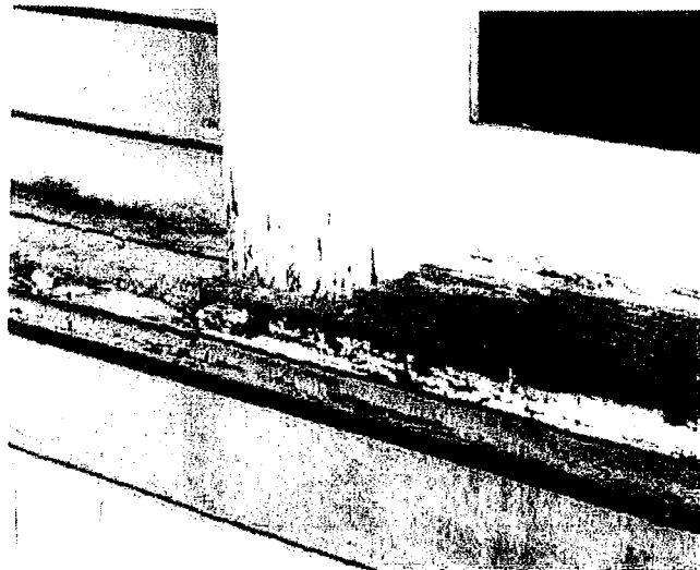
Fig. 4 Paint films wear unevenly depending on exposure and location. Exterior locations which are susceptible to accelerated deterioration are horizontal surfaces such as window sills. These and similar areas will require repainting more often than less vulnerable surfaces. In the case of this window sill where paint has peeled off and adjacent areas have cracked and alligatored, the paint should be totally removed. Prior to repainting, any weathered wood should be rejuvenated using a solution of 3 cups exterior varnish, 1 oz. paraffin wax, and mineral spirits/paint thinner/or turpentine to make 1 gallon. Liberal brush application should be made. This formula was tested over a 20-year period by the U. S. Department of Agriculture's Forest Products Laboratory and proved to be just as effective as water-repellent preservatives containing pentachlorophenol. After the surface has thoroughly dried (2-3 days of warm weather), the treated surface can be painted. A high quality oil-base primer followed by two top coats of a semi-gloss oil-enamel or latex-enamel paint is recommended. Photo: Baird M. Smith, AIA.
